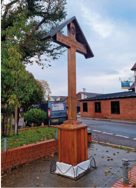
War Memorial renovation.
